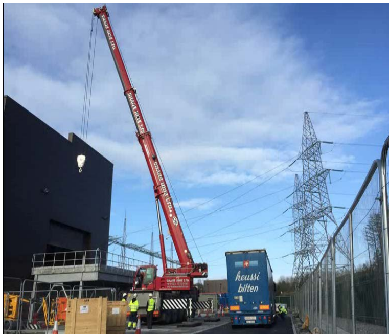
Delivery of switchgear
