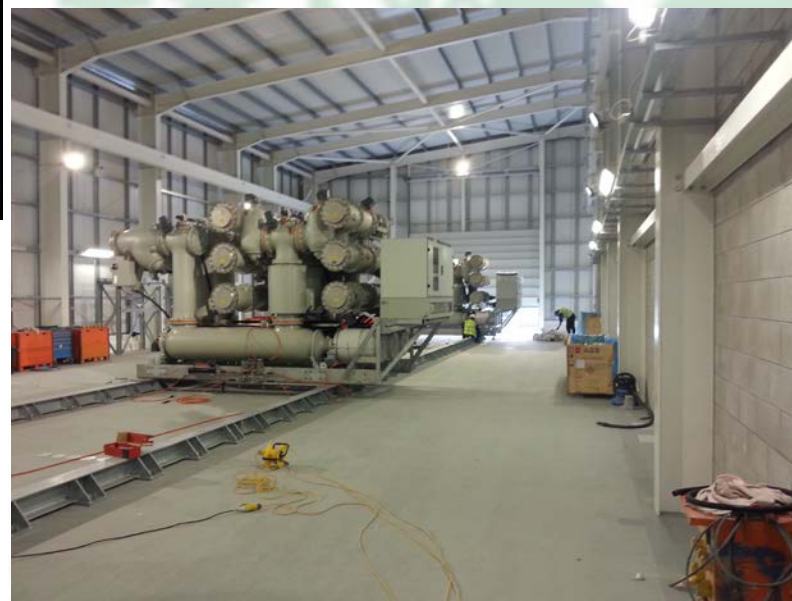
Switchgear being moved into position
