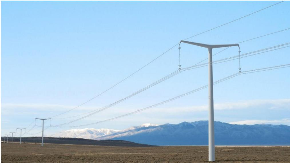
Figure 7 modern pole tower structure for HVDC Transmission (courtesy of Bystrup of Copenhagen)
