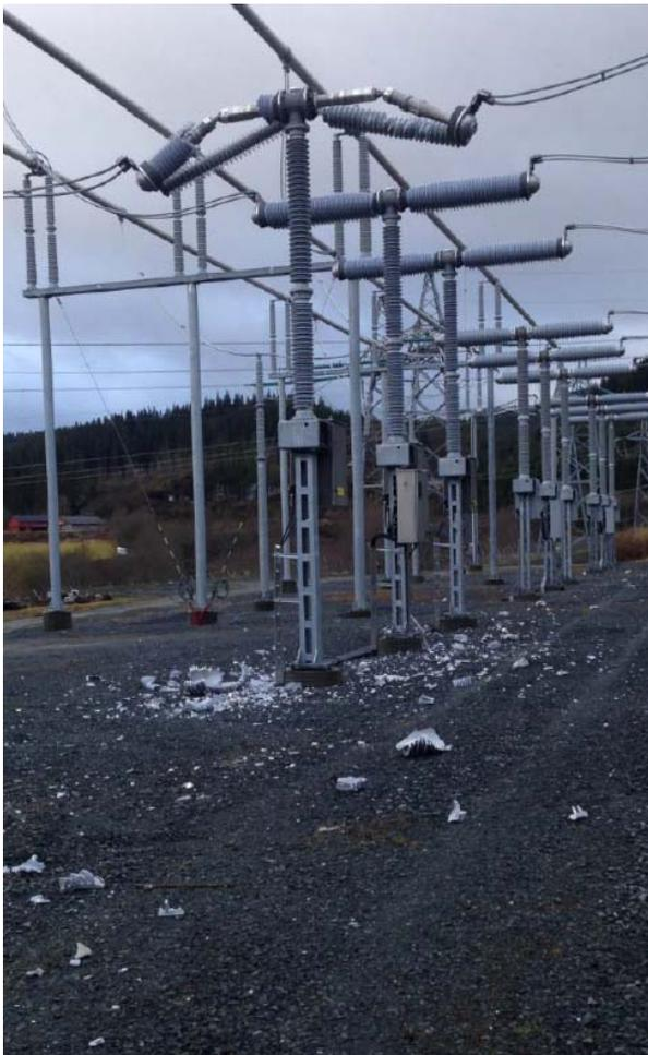
**Figure 1: Fragmentation of 420 kV porcelain insulated circuit-breaker.**
