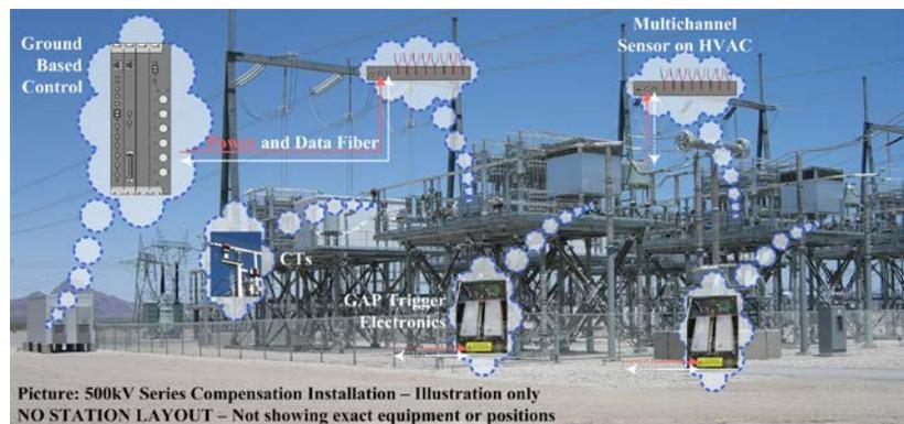
Figure 10: Schematic illustration of HOM7 for (U)HVAC SC application
