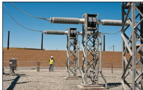
Figure 2: Non-conventional CT with insulation (180kV)
