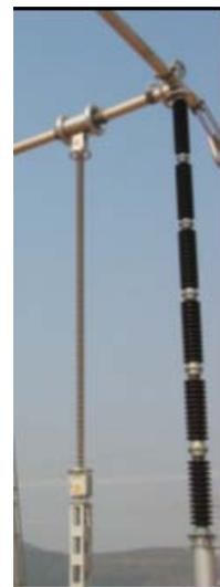
Figure 6: Shunt for  $800\text{kV}_{\text{DC}}$
