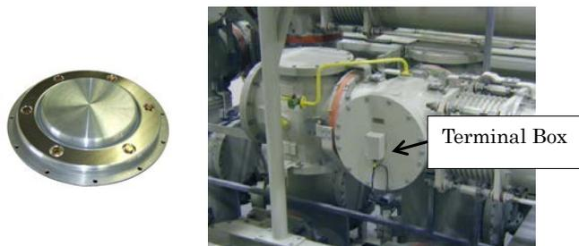
Figure 2 Internal PD coupler and terminal box
