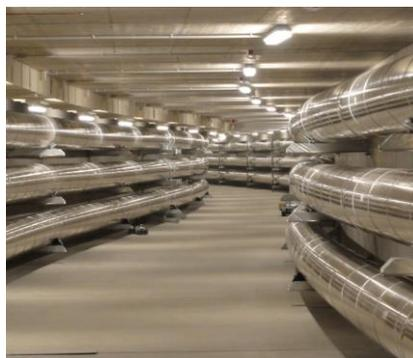
**Fig. 8:** Langwied tunnel with two three phase AC systems, 420 kV, 2300 A
