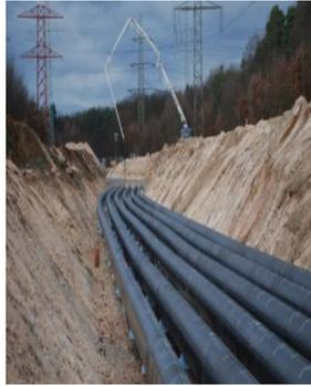
**Fig. 7:** Kelsterbach two three phase AC systems directly buried of 420 kV and 2750 A
