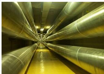
**Fig. 6:** Palexpo tunnel with two three phase AC systems, 300 kV, 2000 A
