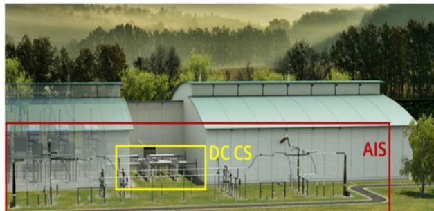
**Fig. 12:** Space saving at the converter station with DC Compact Switchgear (DC CS)
