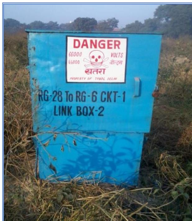
Fig-11 Above the Ground Link Box
