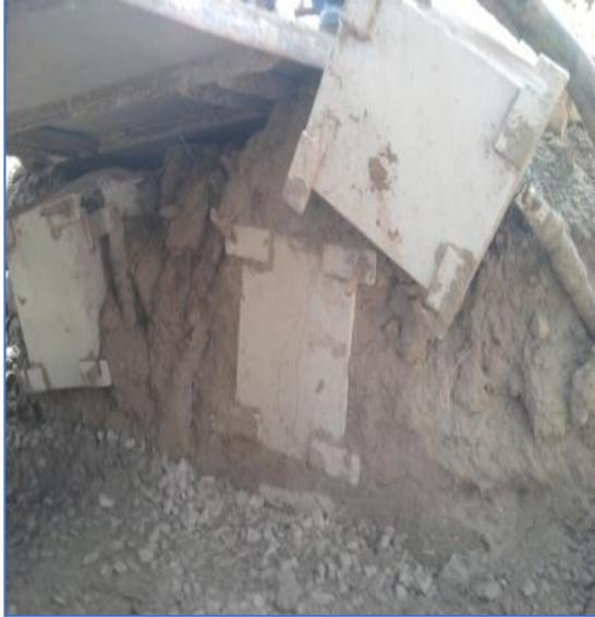
Fig-8, Damaged Link box
