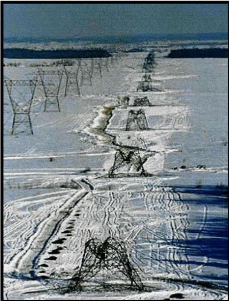
Figure 2 – A 735kV Line Cascade
