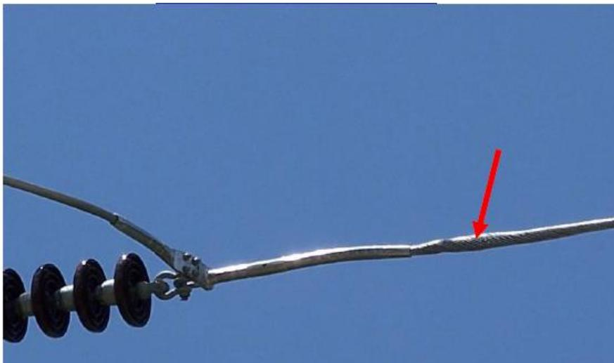
Figure 5 – Bird-caging of Annealed Aluminum Conductor after Compressing Dead-end
