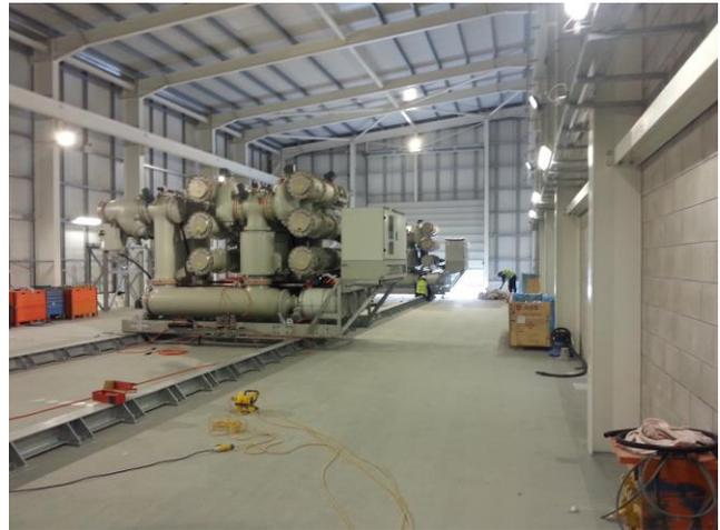
**Figure 7: Switchgear being moved into position**
