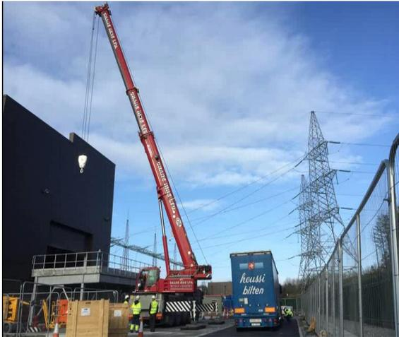
**Figure 6: Delivery of switchgear**
